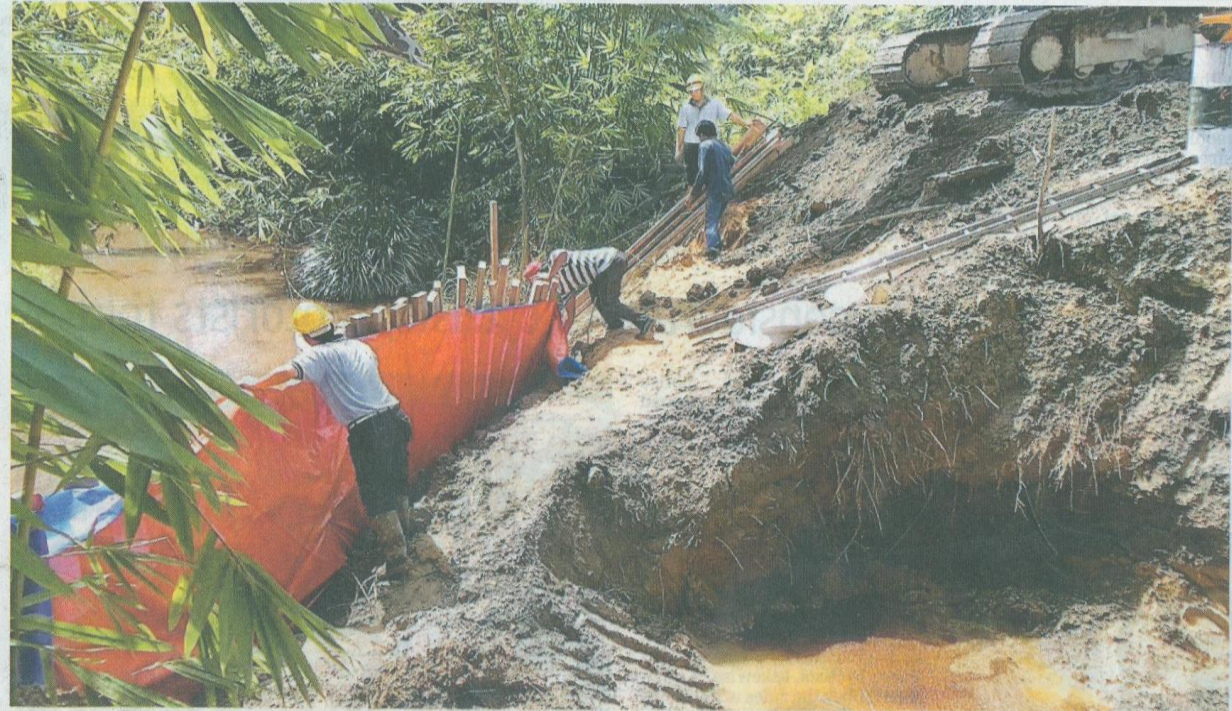
MITIGATION MEASURE: Reinforced trench being dug to collect the leaked diesel and prevent it from seeping into the river
